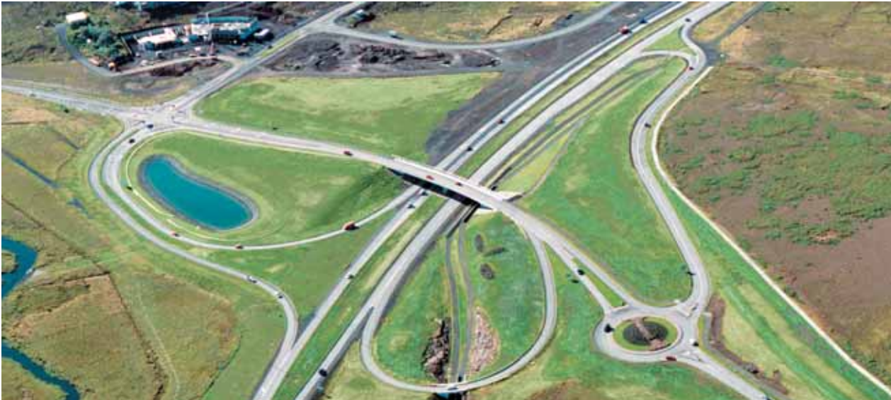
Hringvegur road, flyover connection at Víkurvegur road
