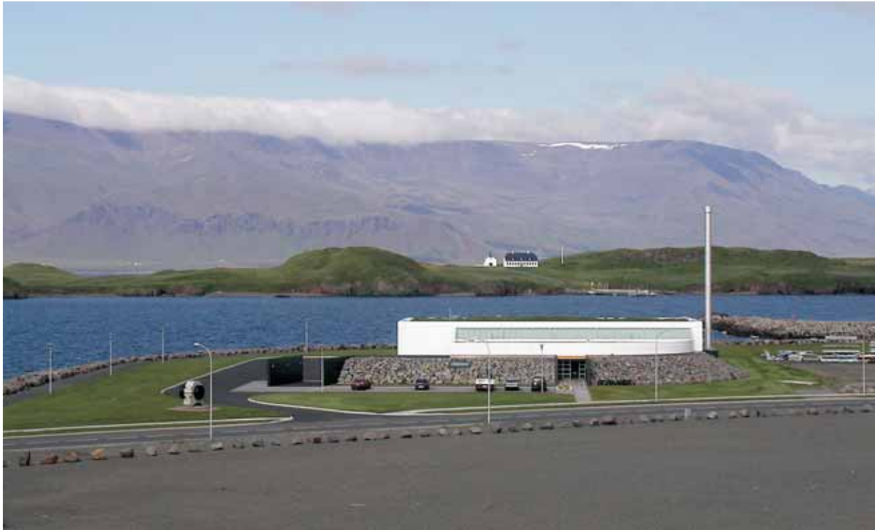
Waste water treatment plant at Klettagarðar, Reykjavik
