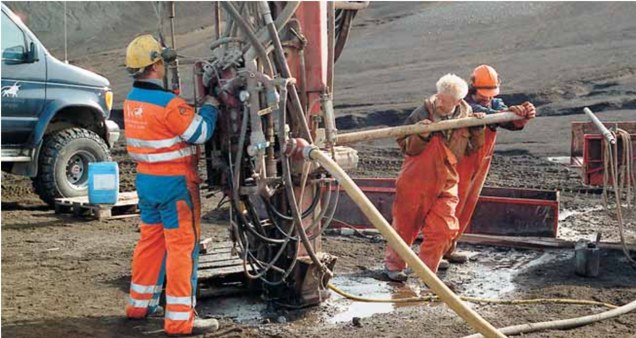
Core drilling at Langisjör
