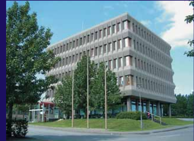
Former head office of Reykjavík Energy
