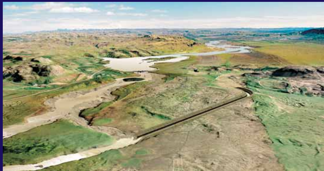
Hvammur Hydropower Plant, one of the options in harnessing Neðri-Þjórsá River (3D visualization)
