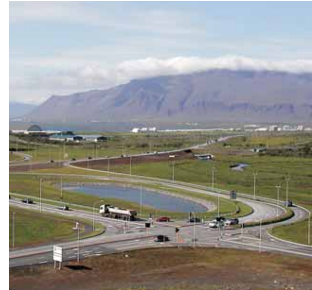
Run-off water settling pond at Hringvegur/Vikurvegur road intersection Photo: Almenna
