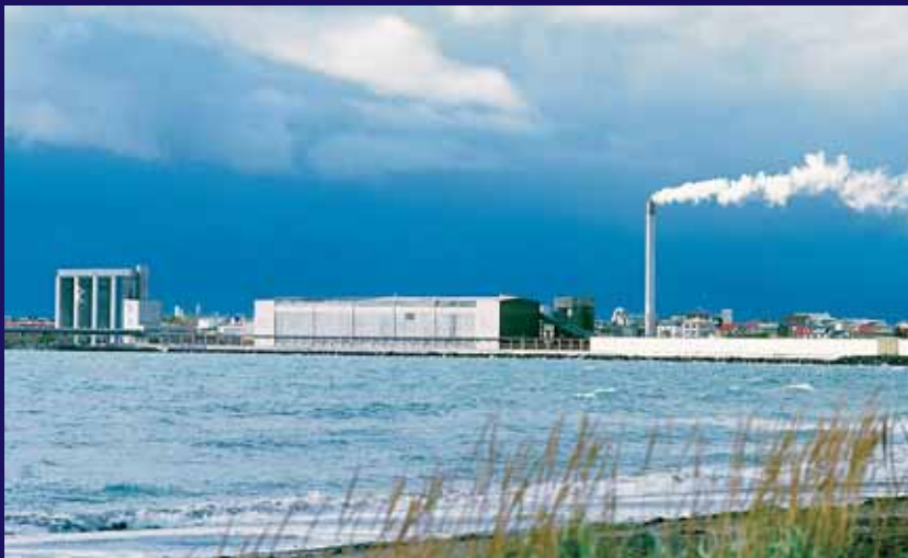
Iceland Cement in Akranes
