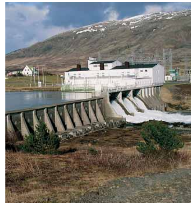
Írafoss Hydropower Plant
