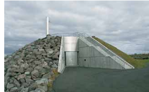
Waste water pumping station in Garðabær
