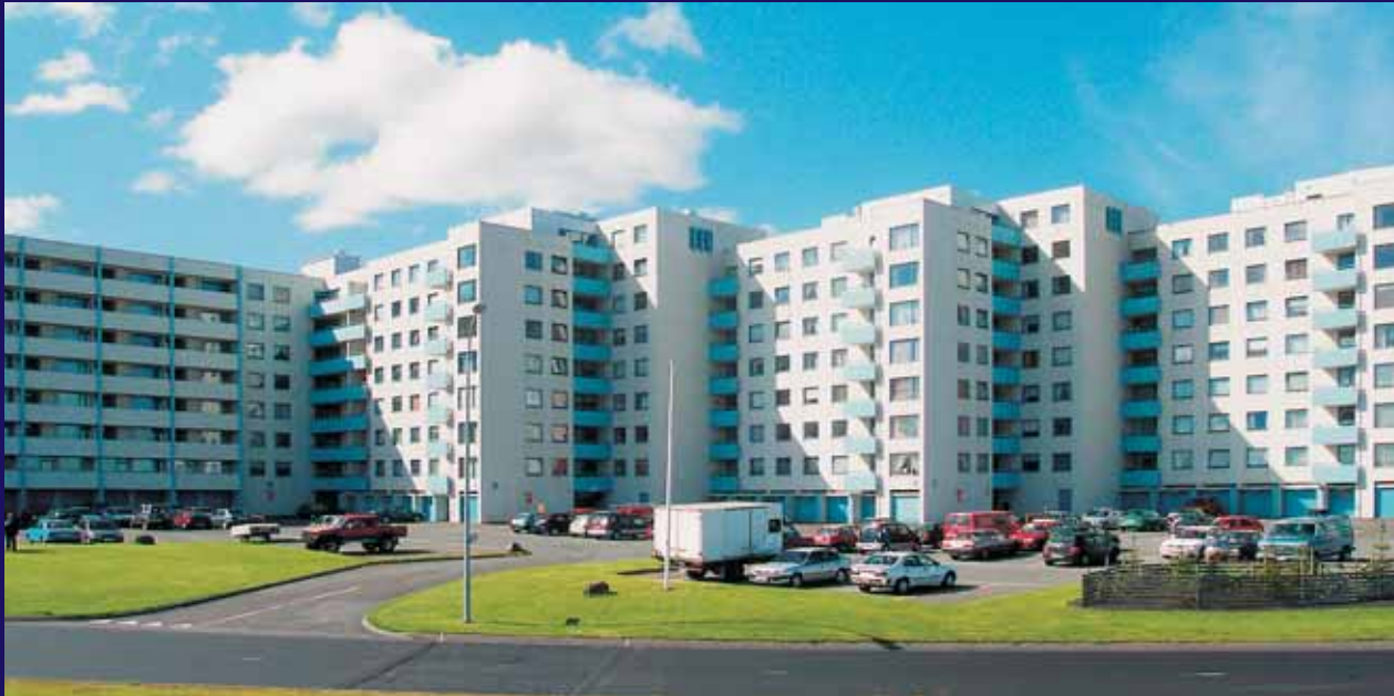
Apartment houses at Asparfell 2-12 in Reykjavík
