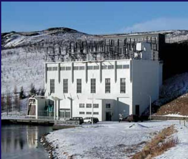
Steingrimsstöð Hydropower Plant
